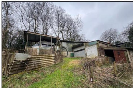
Figure 3: Photograph of the existing buildings on site
